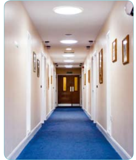
Corridor at the Brain Rehabilitation Centre, Birmingham, lit entirely by SunPipes.
