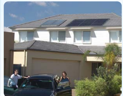
Grid Connected solar installation Sydney, Australia.
