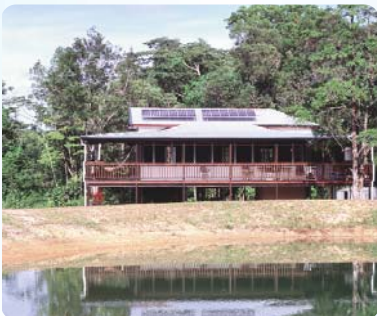
Remote Area (RAPS) installation, Daintree QLD, Australia.
