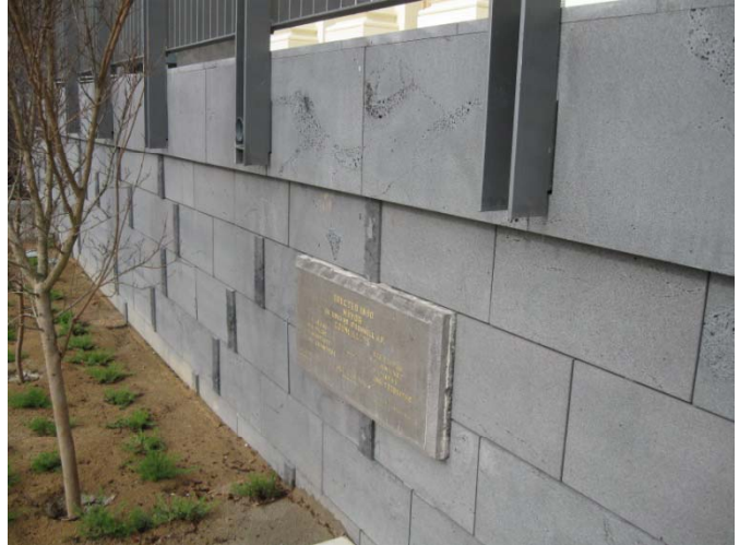
Sawn Cladding St Kilda Town Hall
