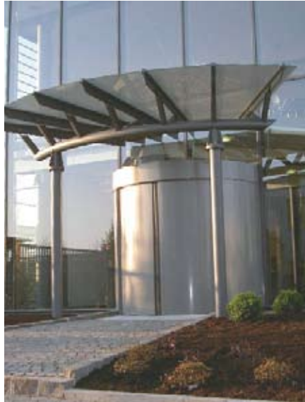
Additional security - four-wing revolving door with night shutters
