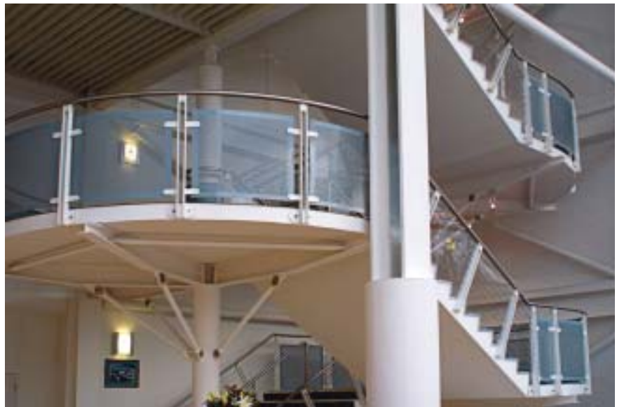
Balustrade infill panels with unperforated margins
