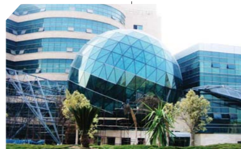
Oncology Hospital (Egypt) Sunergy Green
